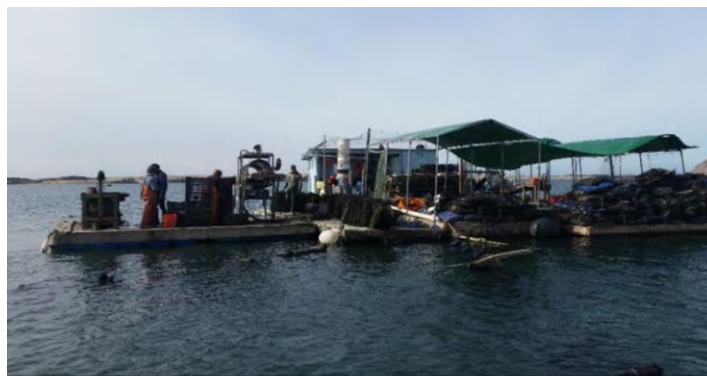
Photo of MBOC's current work barge to be removed and replaced. Photo by: MBOC
